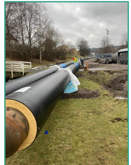
HDD SECTION OF THE JÖNKÖPING ENERGI EXPANSION PROJECT
