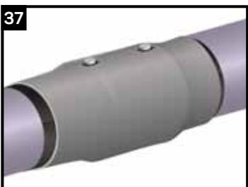
Visually inspect the completed casing. **Ensure that the ends of the CSC are completely shrunk down.** To double seal the foaming hole use a Canusa Foam Seal - CFS.
