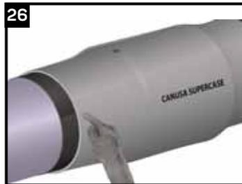
With a gloved finger, press down on the shrunk area to ensure the backing and adhesive are soft. If there are cool spots, the shrink zone should be reworked with additional heat.
