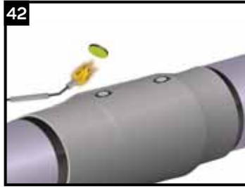
Heat the adhesive side of the CFS with a medium intensity flame until the adhesive becomes glossy (Adhesive will melt).
