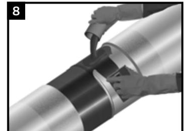
Apply mixed epoxy to a uniform thickness of 4-6 mils (100-150 microns) on all exposed bare metal plus 10mm (0.5") onto the adjacent pipe coating using the applicator pads as supplied or an approved tool. Do not apply the epoxy to the mainline coating.
