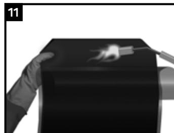
Partially remove the release liner [approximately 1 metre (3') from the edge] from the corner trimmed sleeve edge.
