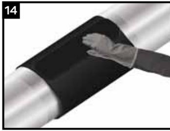
Firmly press the entire closure seal into place. Ensure that the closure is centred evenly over the underlap-overlap sleeve seam.
