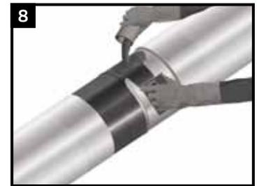
Apply mixed epoxy to a uniform specified thickness of 4-6 mils (100-150 microns) on all exposed bare metal using the applicator pads as supplied or an approved tool. Do not apply the epoxy to the mainline coating. Use a wet film thickness gauge to confirm the thickness.
