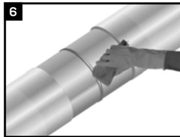
Using a dry, grease and lint-free cloth, wipe clean or air blast the steel and coated areas to remove foreign materials. If necessary, provide additional heat to ensure the surface temperature is 30-50°C (86-120°F).
