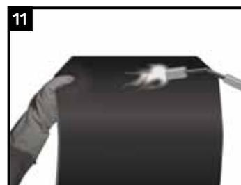
Partially remove the release liner [approximately 0.5 m (1.5') from the edge] from the corner trimmed sleeve edge.
