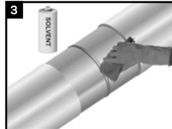
Clean any exposed steel and adjacent pipe coating with a solvent cleanser to remove the presence of oil, grease, and other contaminants.
