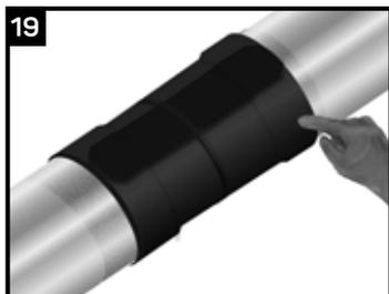
Test sleeve adhesion by gently pulling the edge of the backing back to ensure that the adhesive remains in place and is fully bonded to the factory coating. The sleeve is well bonded when the adhesive and coating remain intimately contacted. If required to improve bonding, additional heat should be applied to the sleeve. Remove protective heat shields when application is completed.
