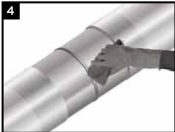
Wipe clean with a lint-free cloth or air blast the steel and pipe coating to remove foreign contaminants. Surface must be clean and dry prior to application of HBE products.
