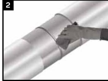
Clean exposed steel and adjacent pipe coating according to SSPC SP 1 to remove the presence of oil, grease, and other contaminants. Ensure that the pipe is at least 3°C (5°F) above the dew point before cleaning.
