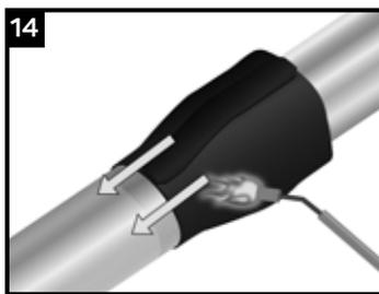
Continue shrinking from the bell of the tyton joint to the sleeve end. Sleeve recovery is complete when it conforms to the pipe.
