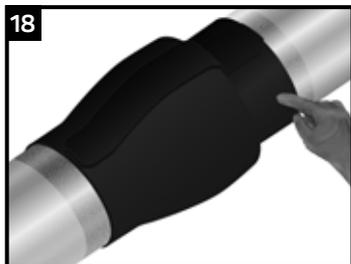
With a gloved hand, press down on the installed sleeve to ensure the backing and sleeve are soft. If there are any cool spots, the sleeve should be reworked with additional heat.
