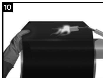
Partially remove the release liner from the sleeve (~15 cm from the edge) and gently heat the adhesive along the underlap with a torch.
