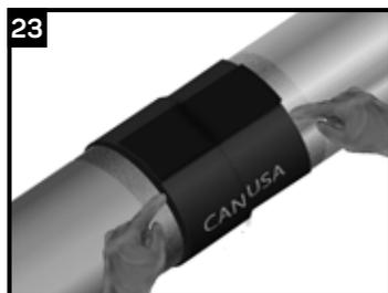
As a final check, ensure that the sleeve follows the entire contour of the surface and that there are no cold spots or burning of the sleeve. **Make sure the edges of the sleeve are not lifting anywhere around the circumference of the pipe.** This can be checked by feeling the edges all around the circumference of the sleeve. If there is edge lifting, the edge should be reworked with additional heat.
