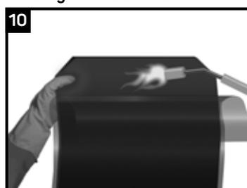
Using the wider sleeve, partially remove the release liner and gently heat the underlap approximately 150mm (6") from the edge. Depending on the TBK directional drill kit, a release liner may or may not be present.
