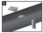
Using a grease and lint-free rag, clean the prepared coating with an approved cleaner (i.e. xylol, xylene, trich, Isopropenol, Acetone, MEK, denatured alcohol) to remove the presence of oil, grease and other contaminants. For damages extending to steel, refer to the Polyethylene Repair Products Install Guide for application of liquid epoxy and filler material.
