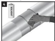
Ensure that the mainline coating edges are beveled to 30°. If there is the presence of oil, grease, or other surface contaminants; clean the exposed steel and adjacent pipe coating with a solvent cleaner.
