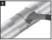
Using a dry, grease- and lint-free cloth, wipe clean or air blast the steel and coated areas to remove foreign materials
