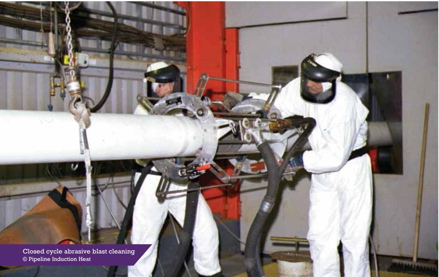
Closed cycle abrasive blast cleaning
