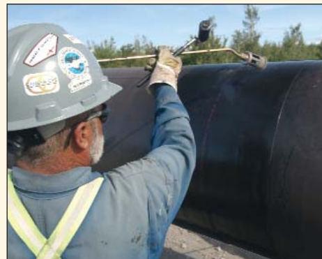
Onshore application of heat-shrinkable sleeves.
