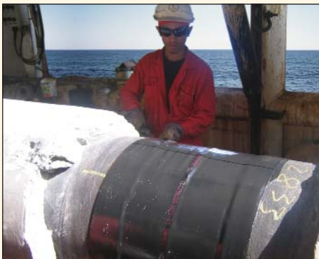
Offshore application of heat-shrinkable sleeves.
