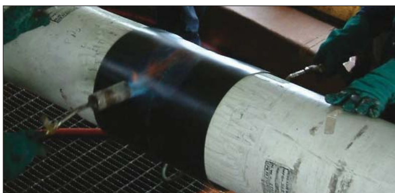
Figure 5. Polypropylene shrink sleeve is applied on an offshore line.
