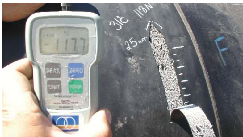
Figure 4. Peel test of shrink sleeve is performed over the mainline coating.
