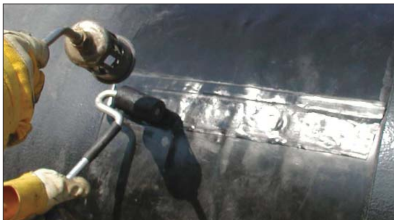
Figure 3. Heat-shrink sleeve applications are installed using hand-held torch and roller.
