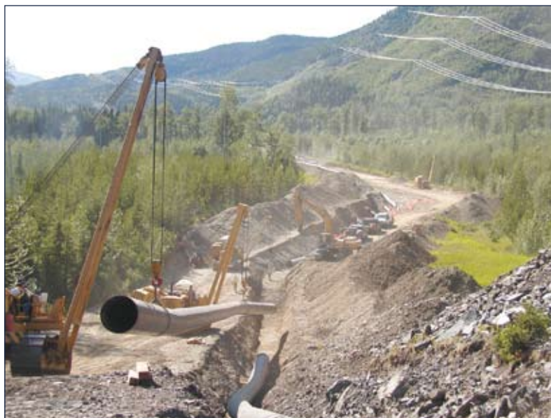
Figure 4. Pipeline construction in aggressive conditions.
