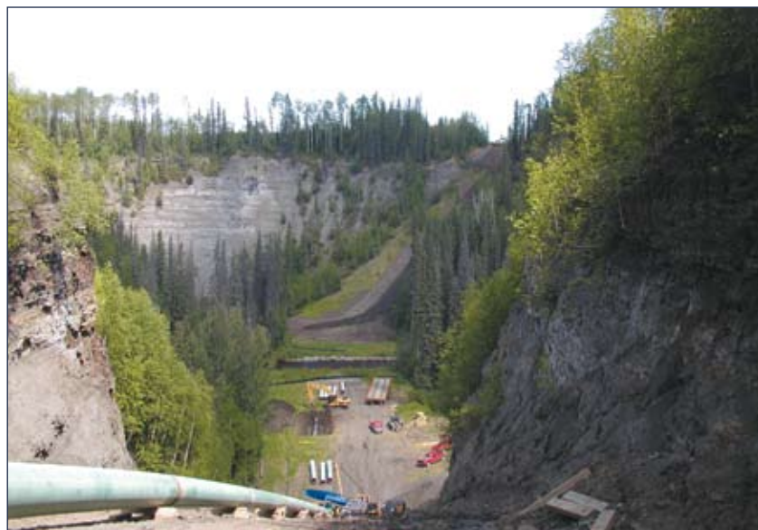
Figure 6. Terrain creates construction challenges.
