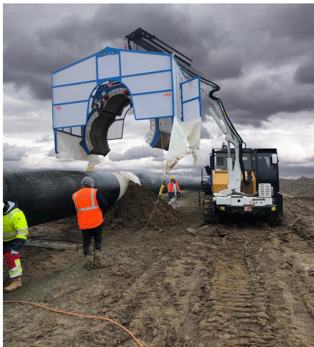
Figure 2. IntelliCOAT with clamshell design preparing to wrap around a large diameter pipeline.
